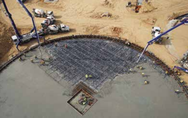
EARTHWORKS & CIVIL WORKS
